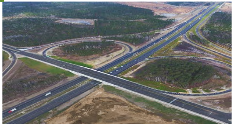
I-26 NEXTON INTERCHANGE
